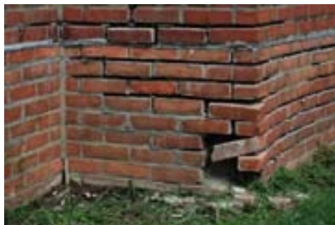
A before picture of the south terrace
