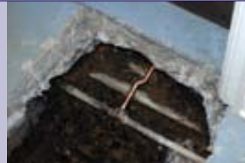
We had to break through the concrete floor to find the water leak below
